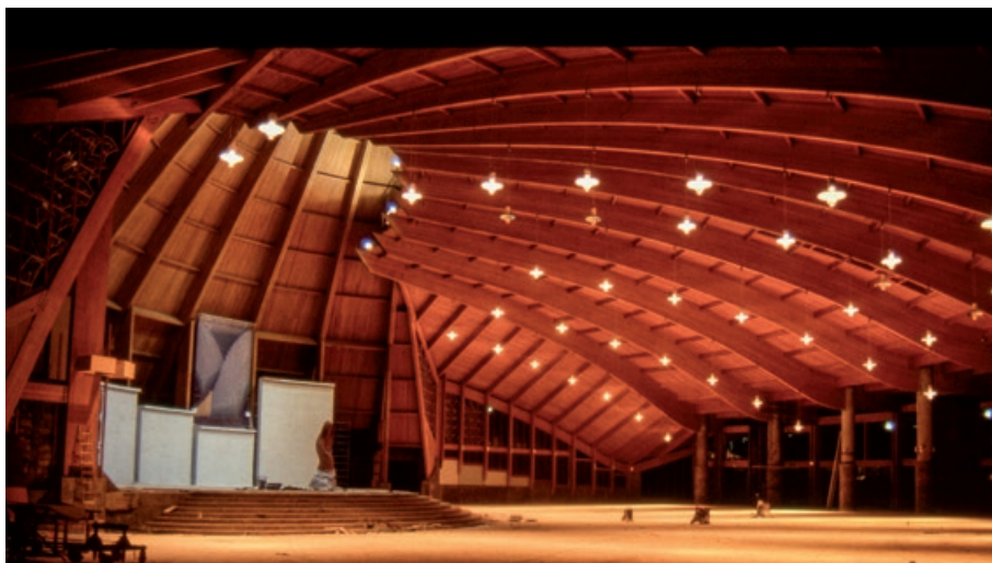
Glued laminated indoor structure at the Mary Queen of the Apostles Basilica in Yaoundé (Cameroon). Photo J. Uhalde, UBC.
