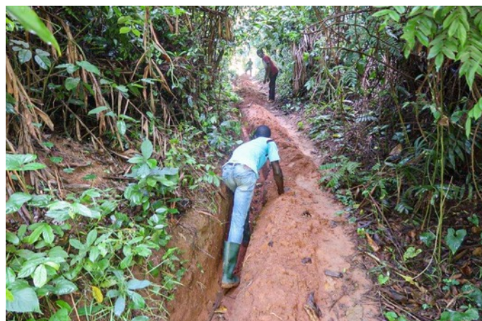
Installing the optic fiber © Luis Arranz
