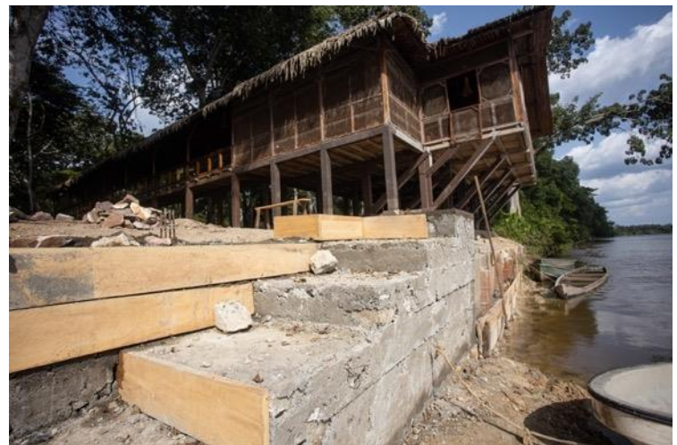
The future existing pier ©Nuria Ortega
