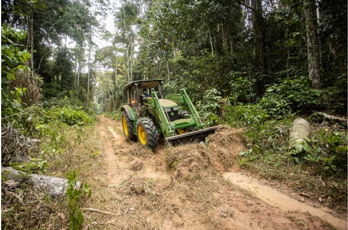
Repairing the roads in the Park © Nuria Ortega
