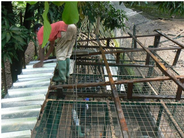
Image 30. Roofing of a Drill satellite cage.
