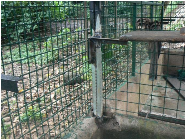
Image 28. Replacement of metal tube in a Drill satellite cage.
