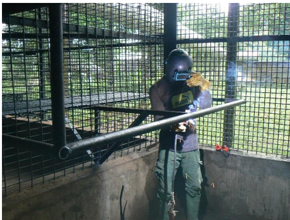
Image 22. Crafting of the framework for the Chimp Mainland platforms.
