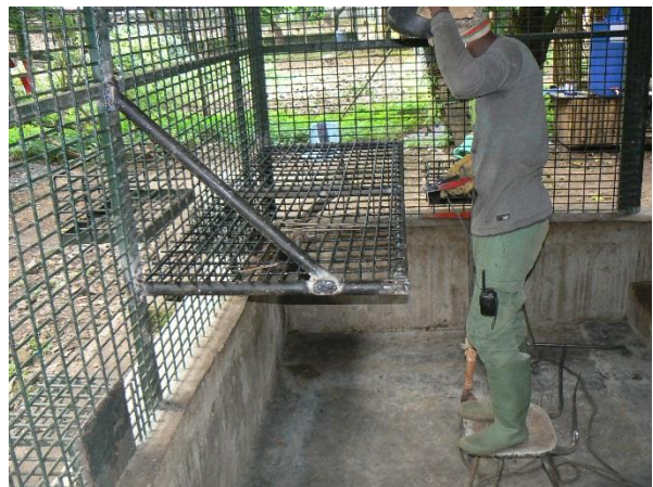
Image 23. Rods mesh installation to form the Chimp Mainland platforms.
