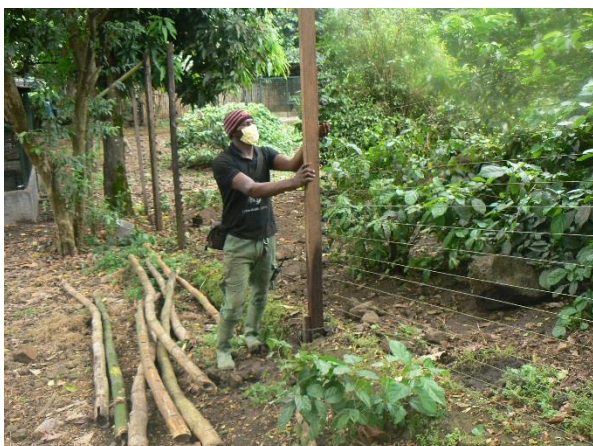
Image 40. Maintenance of the electric fence of the Olive baboon enclosure.
