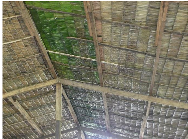
Image 19. Natural raphia palm roof is not only elegant and effective but also helps support a traditional handicraft activity in the local community.
