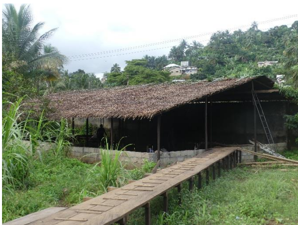
Image 20. Final view of the finished roof of the composting area.
