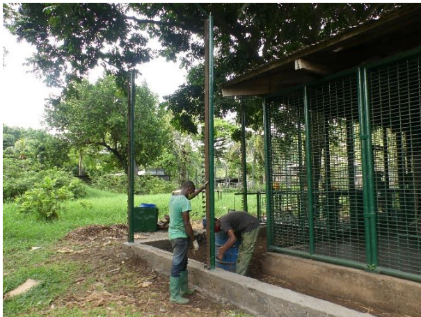
Image 27. Installing ring insulator pole the splitting of the large gorilla enclosure.
