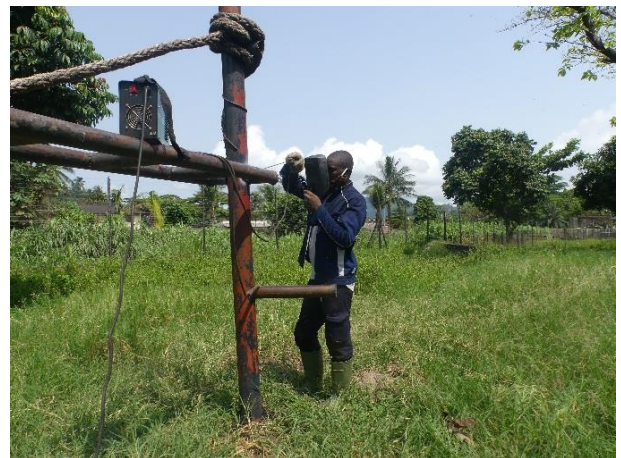
Image 31. Connecting the ladder and welding in the Chimp Island enclosure.
