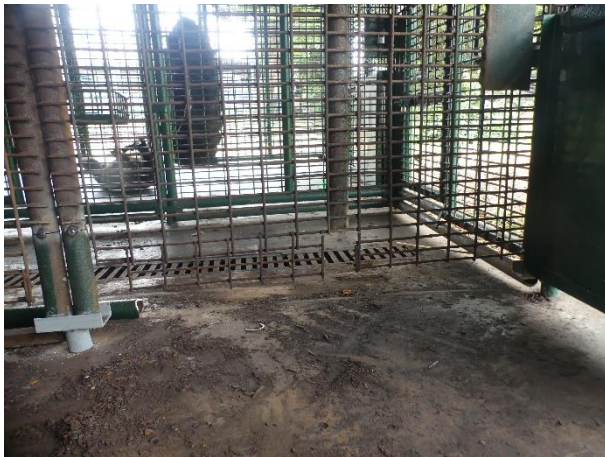
Image 20. The rod mesh in the gorilla 1 night den was fully renovated. We are using 12 mm thick rod to ensure sufficient resistance against the immense power of a silverback.
