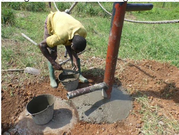
Image 30. Concreting the metal pole of the ladder enrichment in the Chimp Island enclosure.
